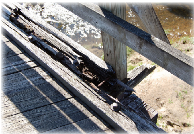
East Blue Creek Bridge damage
