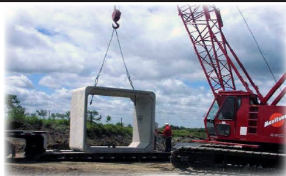
County Home Road culvert placement during the 2004 paving of the Cedar Valley Nature Trail. (Photo Randy Burke)
